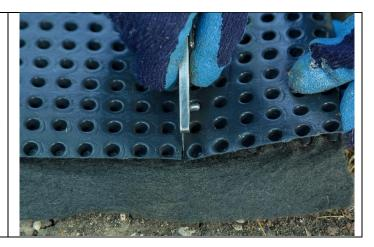
**Step 2:** Remove the top 4 to 6 inches (6 to 9 dimples) of plastic core exposing the fabric.
