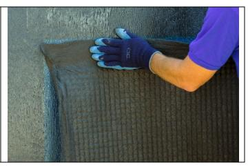
**Step 5:** Working from the top down, apply heavy, uniform pressure to compress the drain board into the adhesive. Be sure to also compress the fabric on the sides of the board into the adhesive. Fabric and plastic core should exhibit a strong initial bond to the adhesive.
