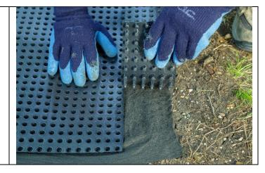
**Step 3:** Apply a full coat (80%-100% coverage) of adhesive across at least the top 4 to 6 inches of the membrane where the drain board will be installed. Use a frame and fill pattern to apply adhesive to the rest of the membrane.
